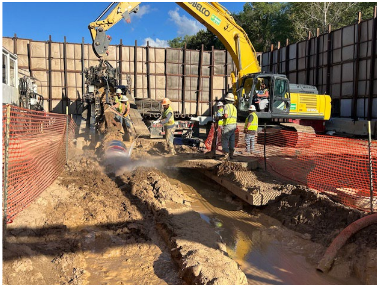
Facing west at HDD P4-1, North Country completed the pull
