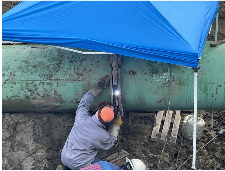
Facing east at MP 31.72, K&K completing mainline tie-in south of 140th Street
