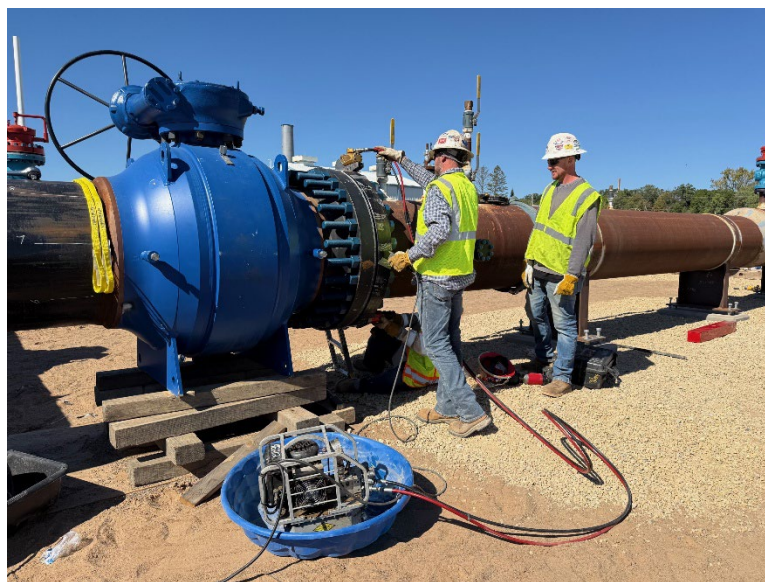
Facing west, view of Otis bolting the valve in place in the Hugo compressor station near MP 0.1
