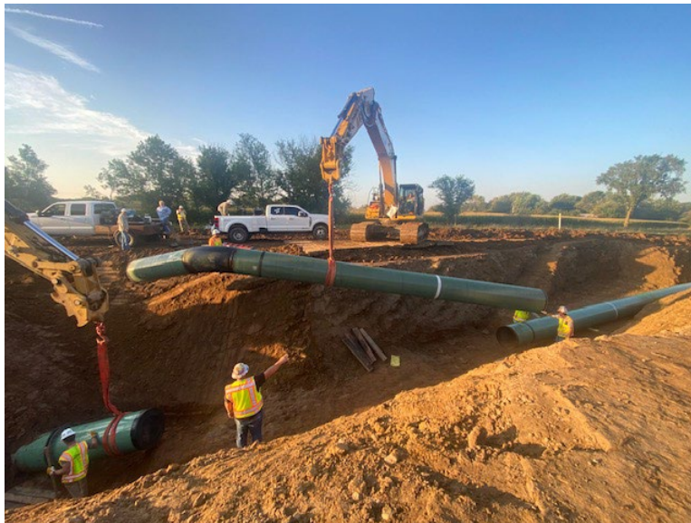
Facing west near MP 1.83, lowering-in ongoing
