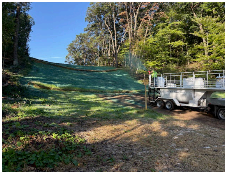
Facing west near MP 2.5, hydroseeding completed
