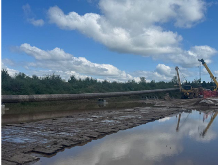
Facing east at HDD P4-5, Mears commenced the pipe extraction
