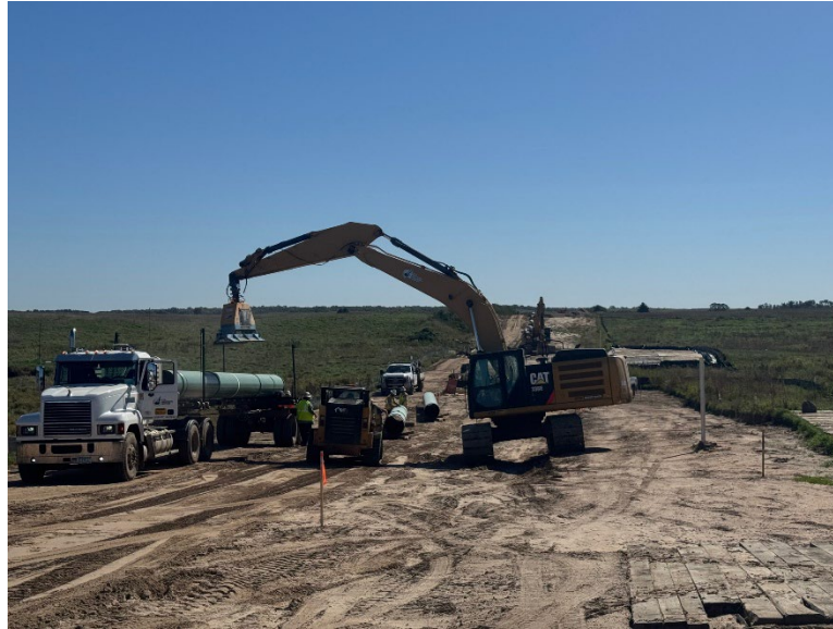
Facing south, view of Otis stringing line pipe near MP 1.18
