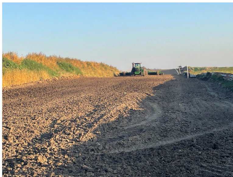
Facing north at MP 31.4, subcontractor for K&K, decompacting subsoil south of County Road 9/135th Street
