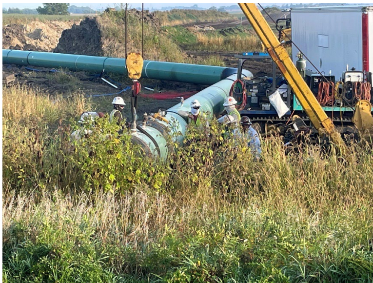
Facing north at MP 31.2, K&K completing installation of test header for E-line extension north of County Road 9/135th Street
