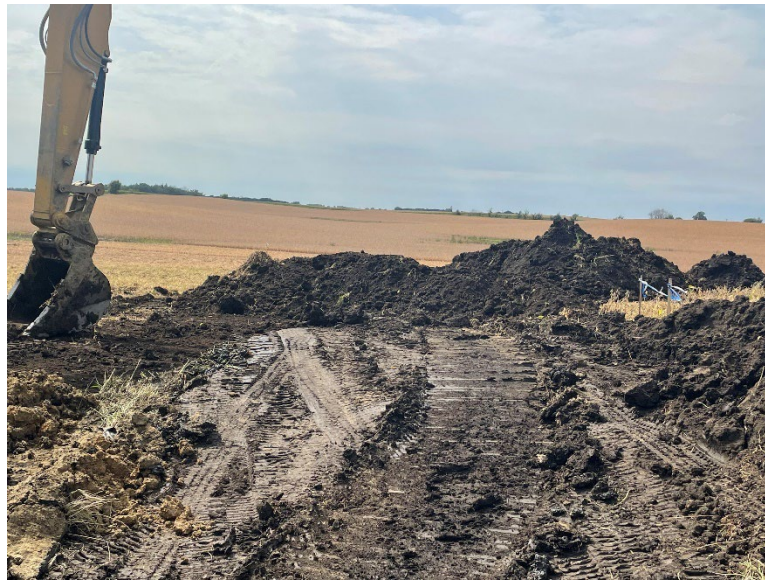
Facing northwest at MP 32.8, K&K removing and stockpiling topsoil for extra workspace north of 140th Street
