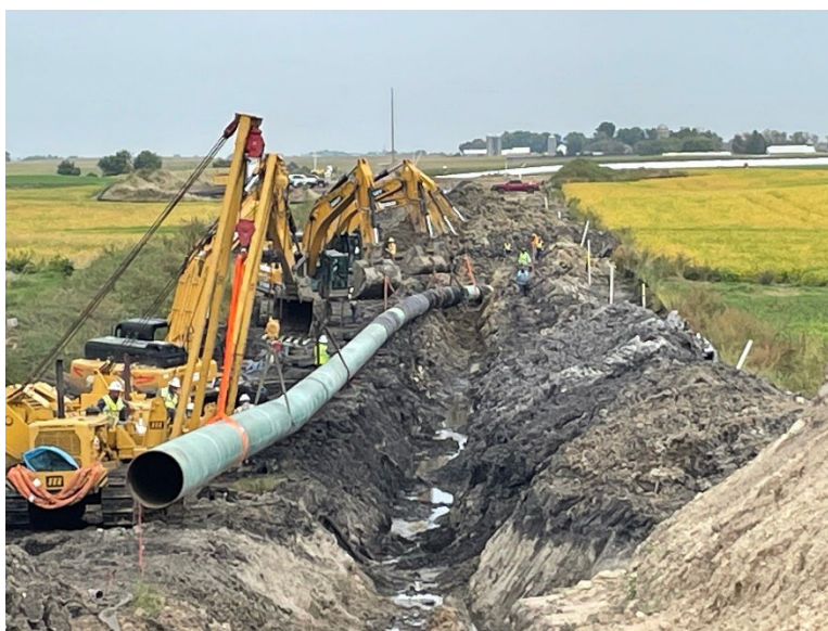
Facing north at MP 32.2, K&K lowering-in mainline pipe north of 140th Street
