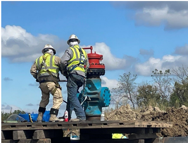
Facing east at MP 34.2, K&K installing valve cap, completing fabrication of D-line tie-in piping
