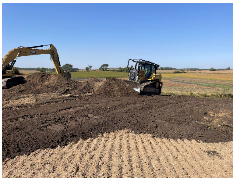
Facing southwest at MP 31.5, K&K restoring topsoil south of County Road 9/135th Street
