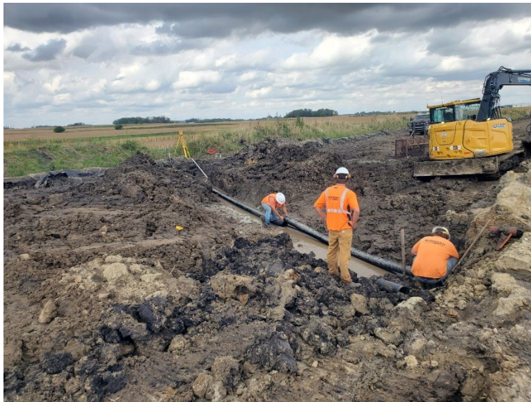
Facing northwest at MP 34.0, Hodgman repairing drain tile south of 165th Street
