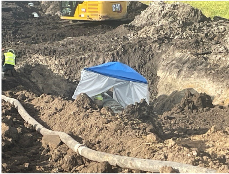
Facing north at MP 31.55, K&K sandblasting and coating mainline trench tie-in south of 140th Street
