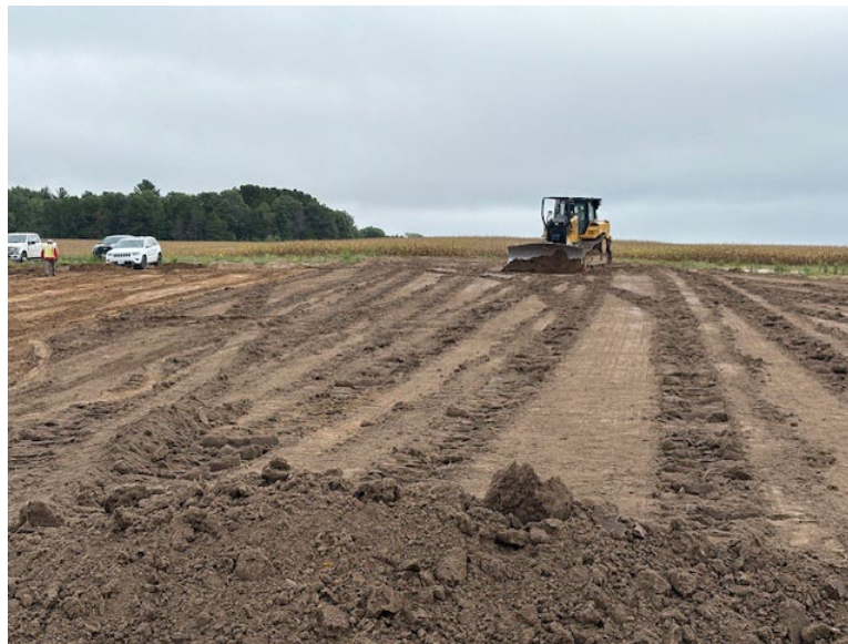
Facing east near MP 3.5, K&K restoring topsoil
